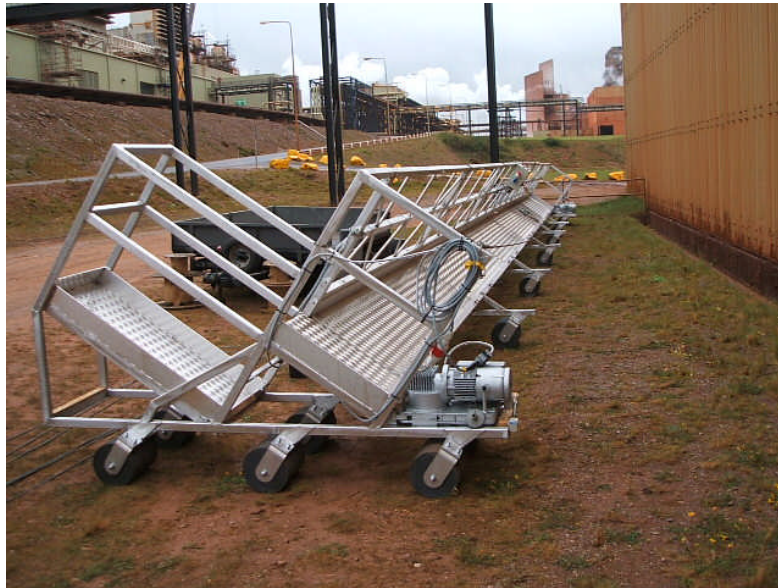
Platform is assembled at ground level before being installed onto the roof.
