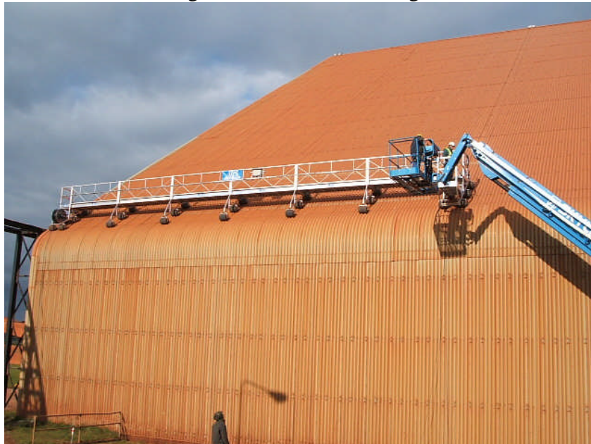
Platform is assembled at ground level before being installed onto the roof.
