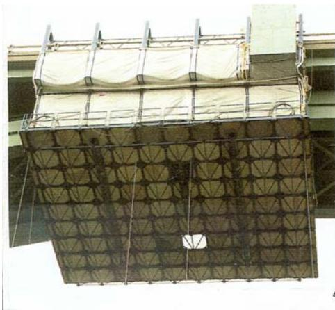
Bridge blasting and painting projects, including all necessary steelwork repairs can be safely and effectively carried out using ALPS Steel Truss Frame or Alloy Space Frame modular suspended access platforms.
