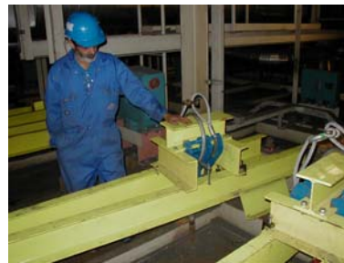
The "Roof" with support steel in place.
