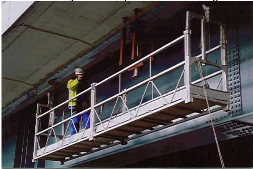
A 6M X 800mm alloy suspended access platform is installed to the new runway beams. The beams and fasteners are examined and proof load tested using the special calibrated jacking system designed by ALPS for this application. The test load can be held in place whilst the fixings are examined.
