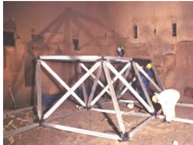
The space-frame is assembled
