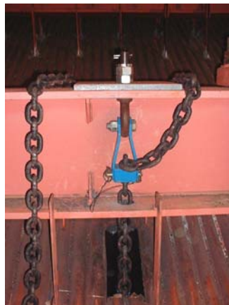
Left: Anchor location above "Attic"
