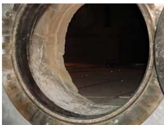
580mm opening into boiler
