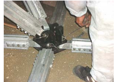
typical lower node and cord
