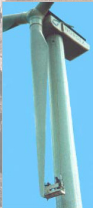
Inspection Cradle suspended from the gondola
