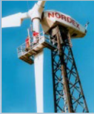
Inspection Cradles during erection of the wind-mill, suspended by a crane
