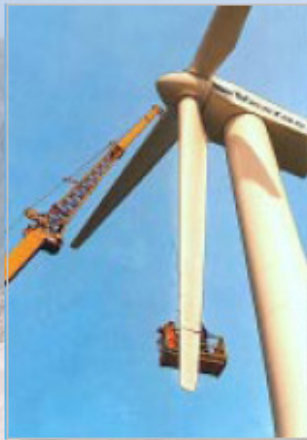
Inspection Cradles during erection of the wind-mill, suspended by a crane
