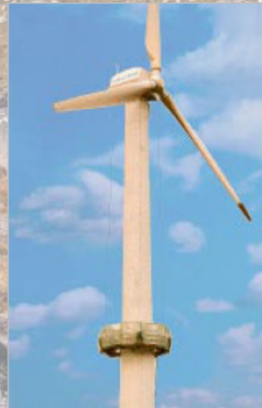
Circular Scaffolding for painting and maintaining the tower shaft
