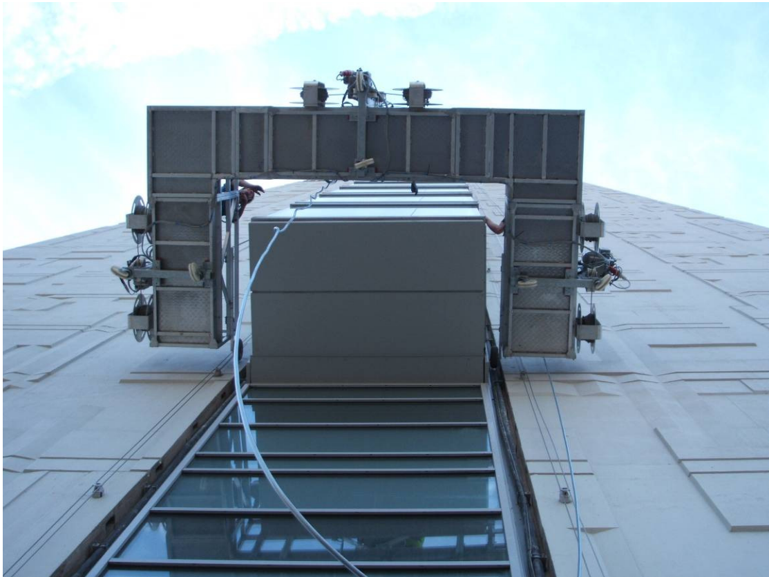
Note: Wire rope guiding system installed
