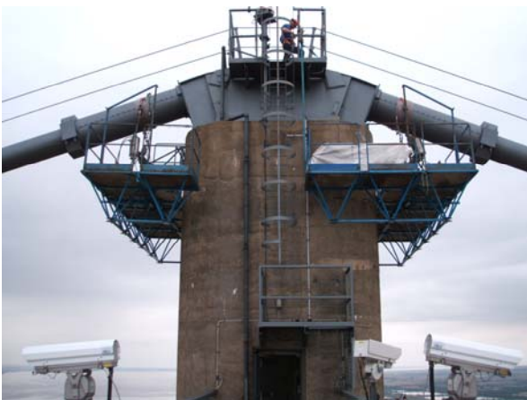
Return sections being installed
