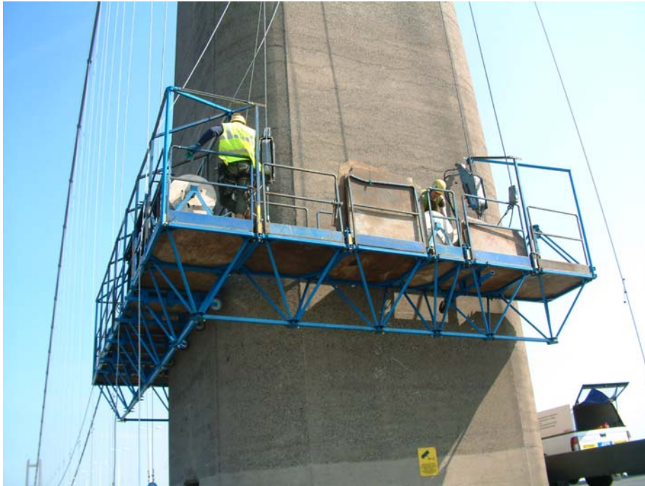
Platform on way up the concrete pylon
