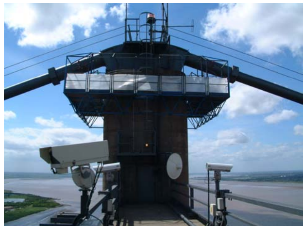
Return sections & sheeting in place
