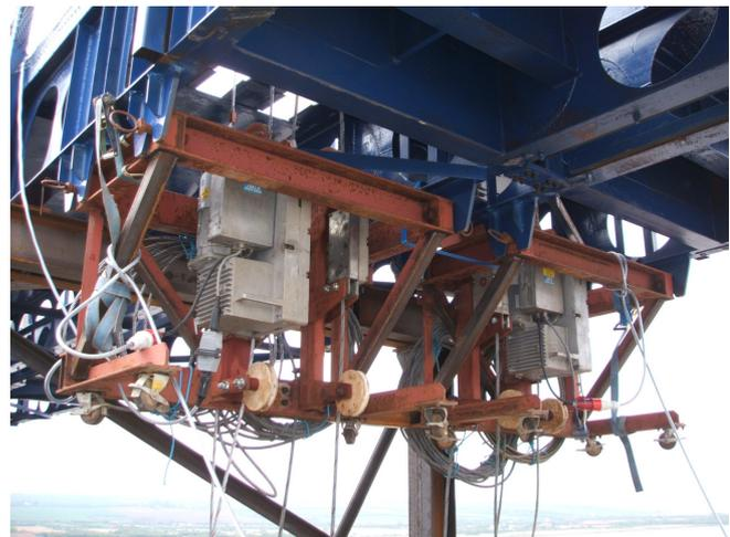
Above: The main cable access platform is installed by ALPS specialist Rope Access operatives using 4 x 3000Kg rope conveying winches and safety devices; right >
