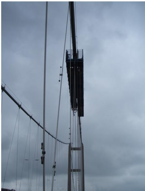
Once ALPS had carried out the lift the man working platform was secured in place and a powered feeder cradle was installed to ensure operatives and equipment could be transported vertically too & from the working platform.
