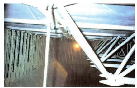
A hinged section is incorporated to enable access to the super-heaters at high level.
