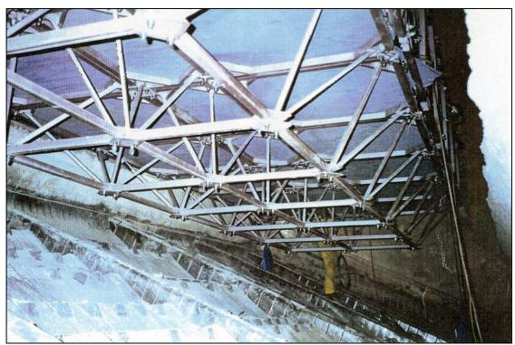
The Steel Truss Frame suspended access platform is quickly assembled and suspended from four access hoists and secondary safety devises.
