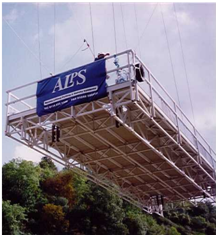
The new gantry is raised from the river.
