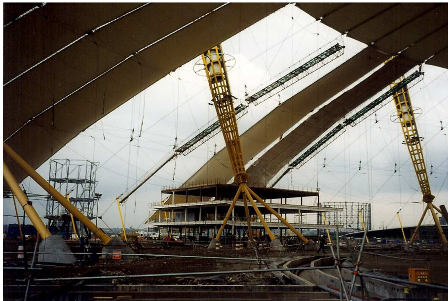
Dome roof with fabric net installation in progress.
