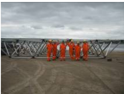
Platform frame is assembled in one shift
