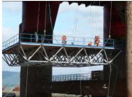
Platforms are raised into place in a few hours
