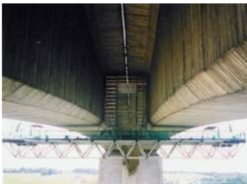
12M Alloy Tower on board main platform
