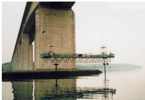
27M Platform lifted from barge and “Going-Up”
