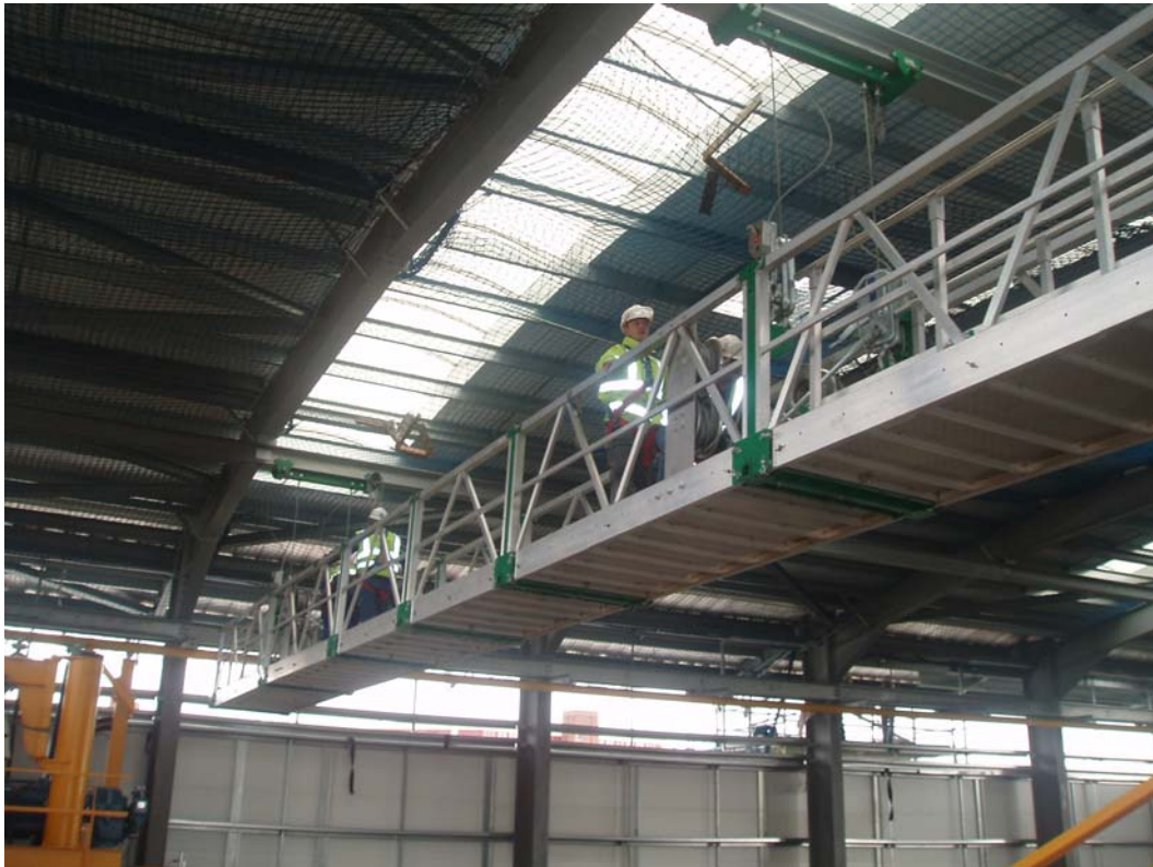
Platform undergoing its initial thorough examination following installation.
