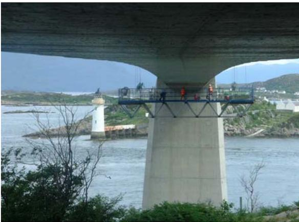
The 14.64M X 4.88M Platform raised from the barge and in place ready for work:
