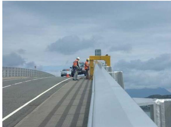
The Mobile suspension stirrups leave the carriageway, foot & cycle path unobstructed:
