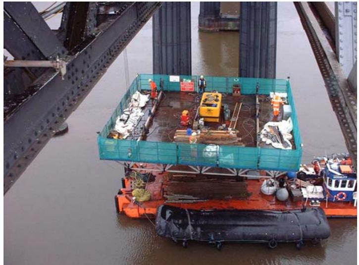
The three large ALPS Underdeck Access Platforms are assembled on the quayside. Each platform is equipped with on board 17Kva generator, 600cfm compressor and other required equipment for the task in hand. The capacity of each platform was 10-Tons.
